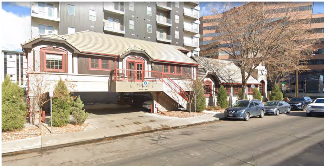
Subject site facing north, on Ellsworth Ave.
