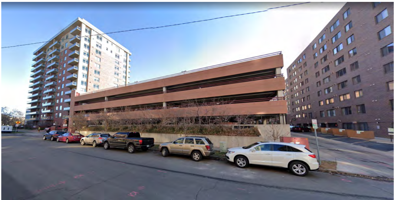
View from the site, looking south (across the street on Ellsworth Ave.)
