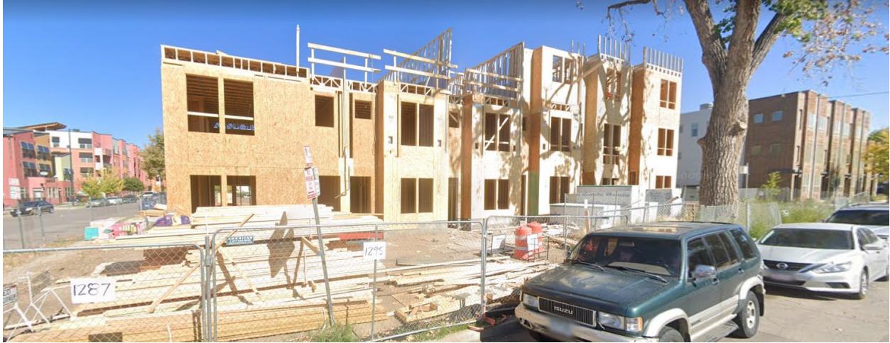
East of site: Looking east from Navajo Street (Source: Google Maps)
