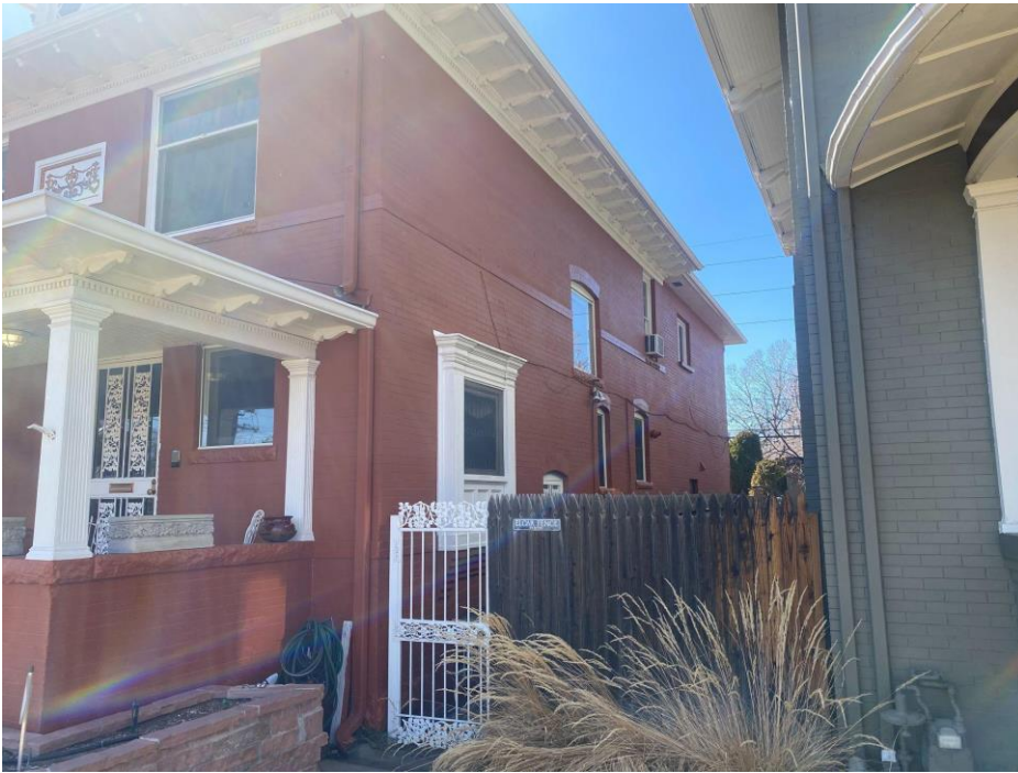
Photo 2. Northeast corner, North elevation.
