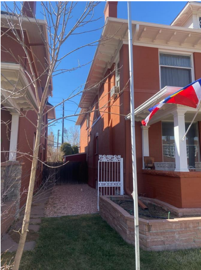
Photo 3. Southeast corner, South elevation.
