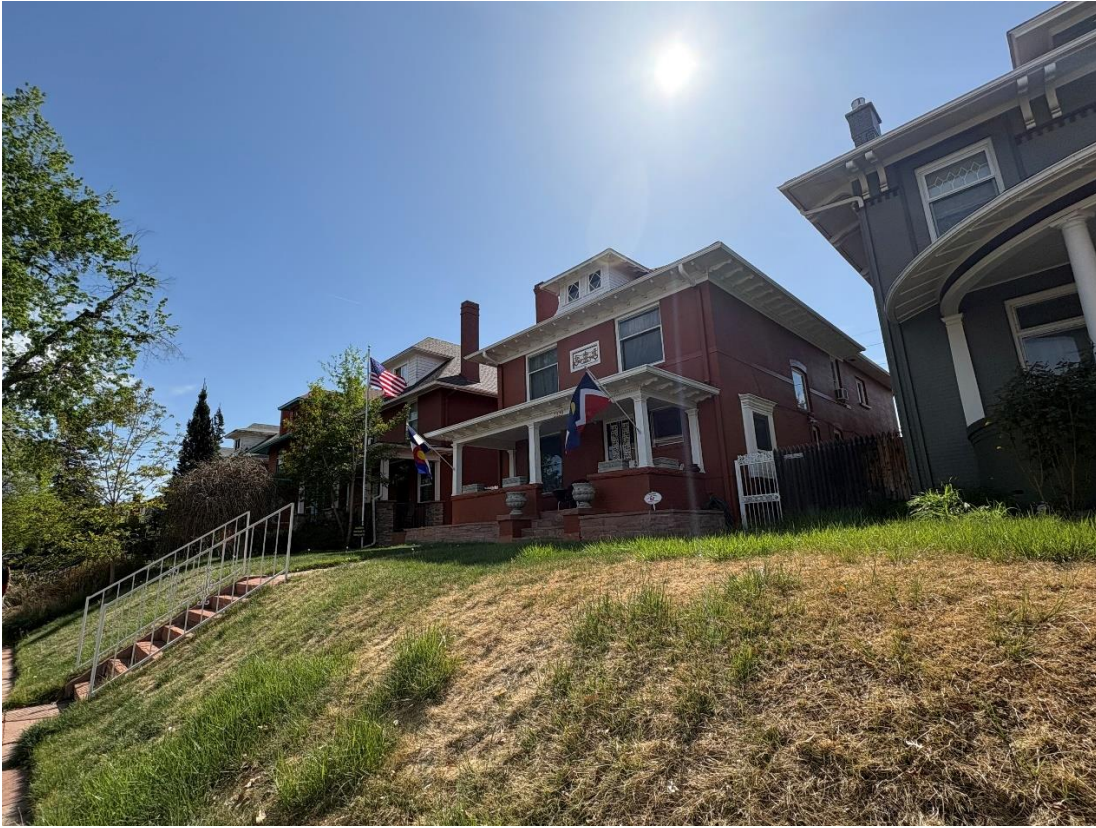
Photo 8. Overview showing east façade and adjacent residences.
