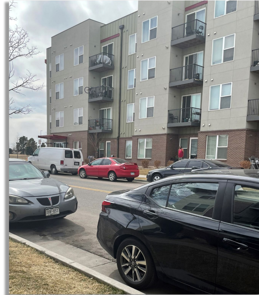
Photo of Park Hill Station multi-family units, north of the site
