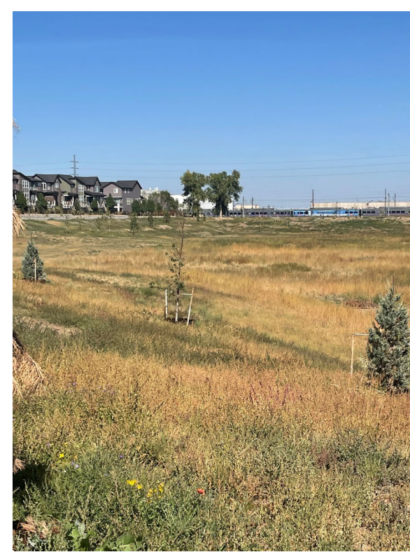
Regional stormwater detention area, Sept. 2021
