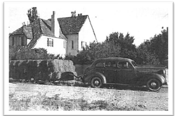
Undated c. 1935 photo of Rear (East) and South Elevations, 2900 S. University Blvd.
