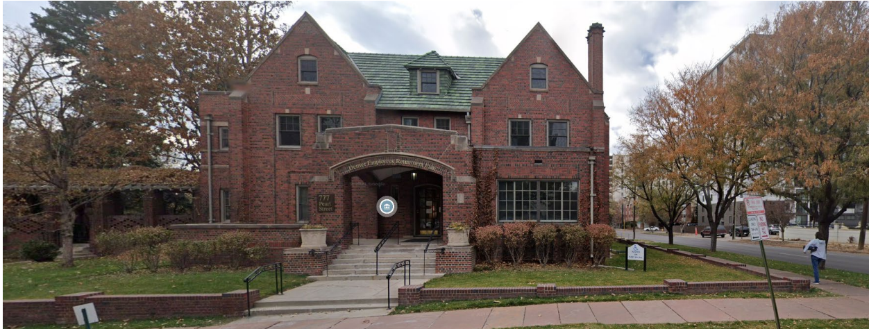
South – DERP Offices (Parcel 1 in PUD 34) from North Pearl Street (Source: Google Maps)
