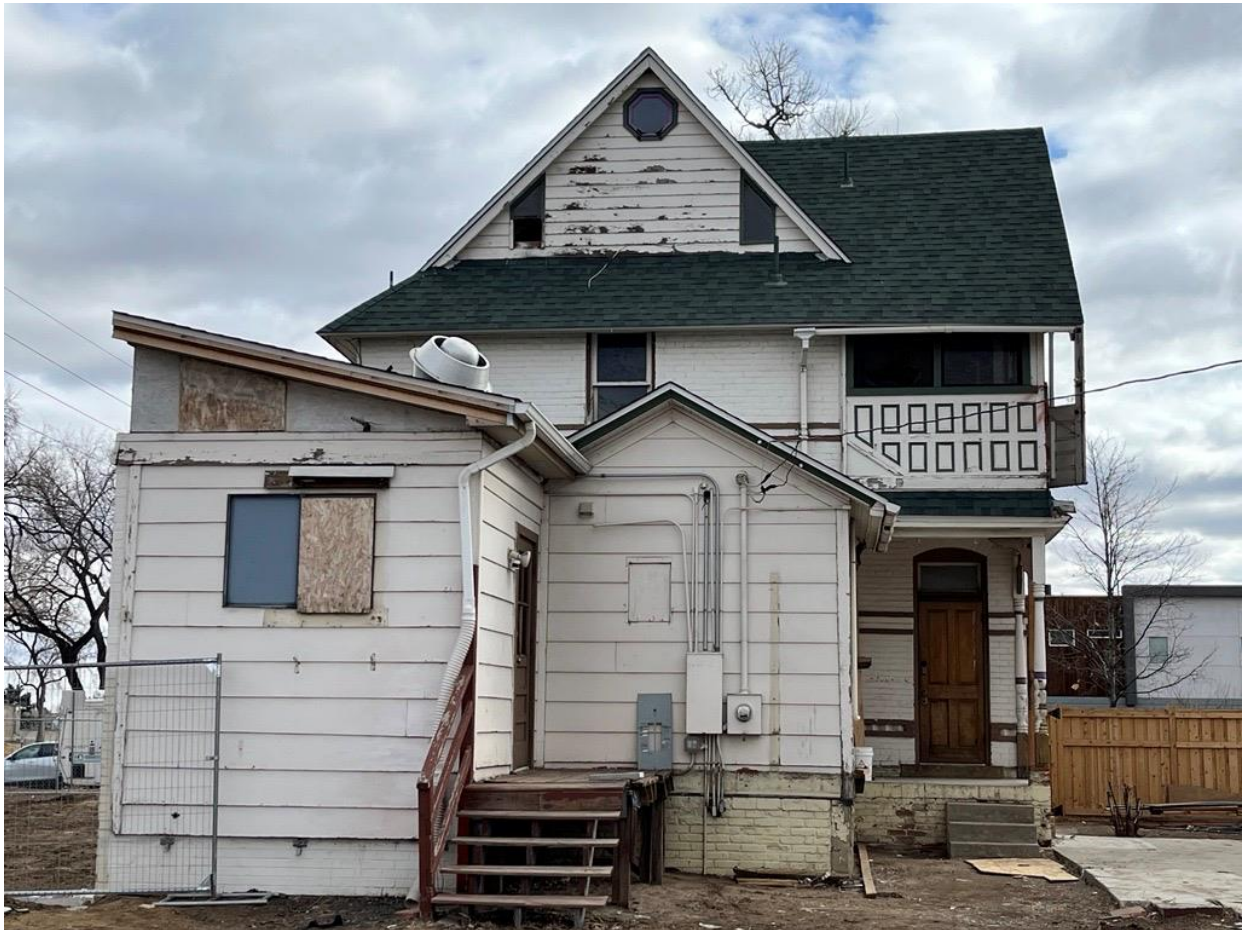
3435 Albion Street, rear facade, with additions
