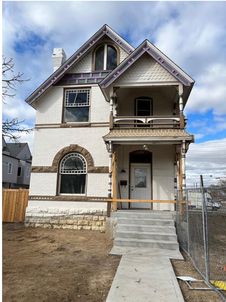
3435 Albion Street, front façade
