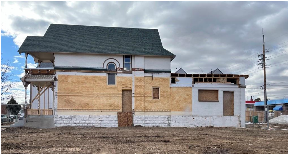
3435 Albion Street, side façade and rear additions
