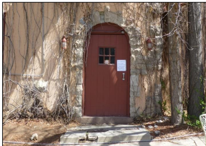
2900 South University Blvd, Window, door, and stone detailing
