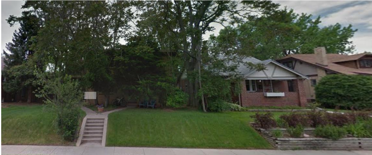
South — from 19 th Avenue looking south
