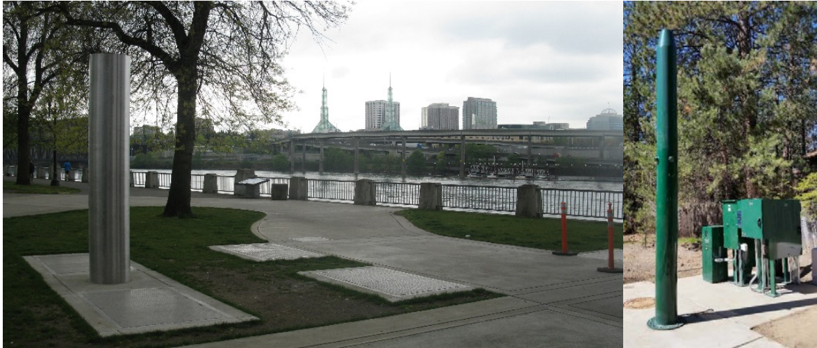
Figure 11- Photos of example stacks for enclosed biofilters.
