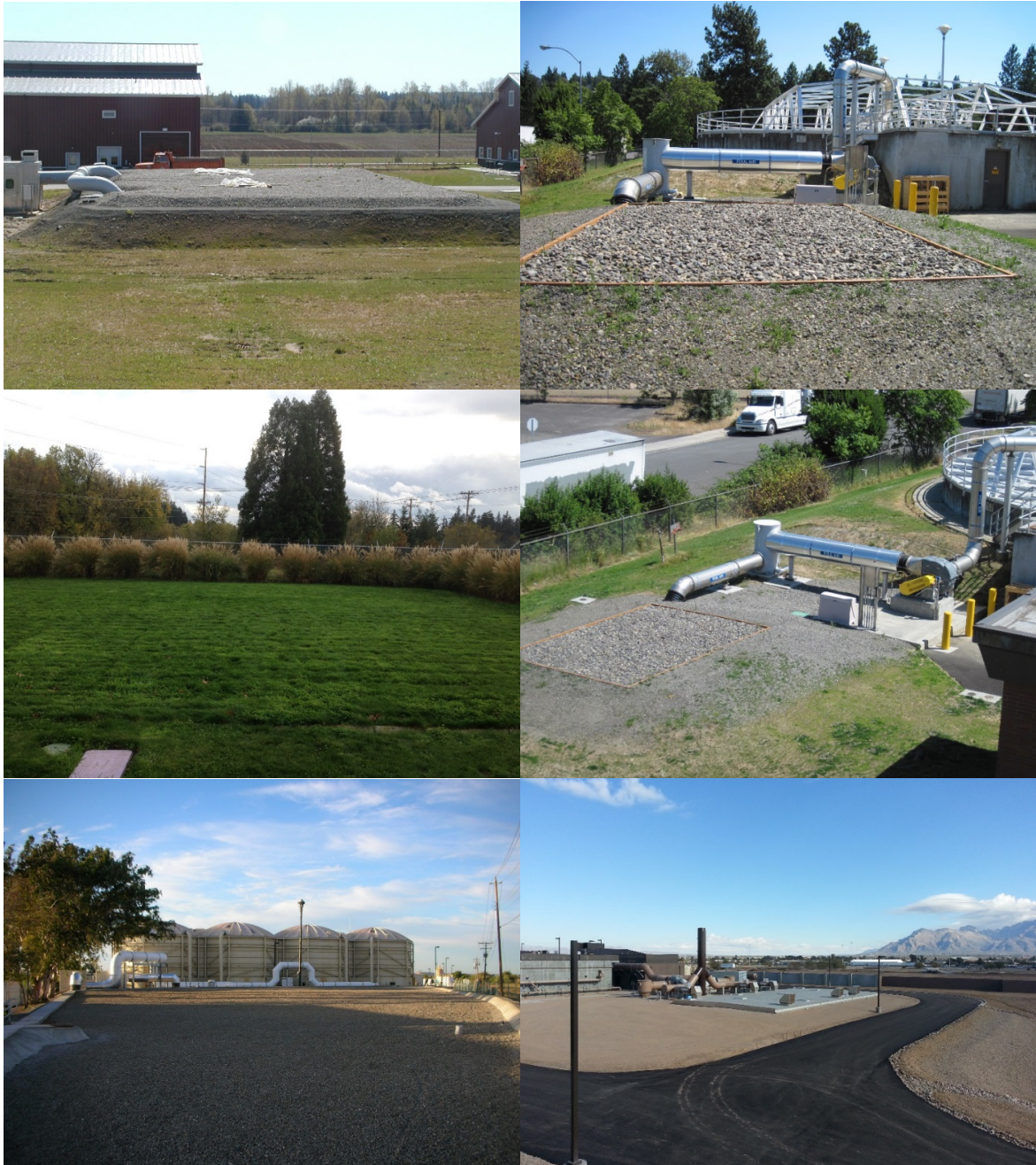
Figure 10 - Photos of example biofilters. These biofilters were designed to blend into the landscape and are provided with a cover, grass or river rock on top and construction with the top flush to grade.
