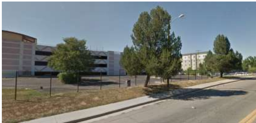
Subject property; surface parking lot; view from Decatur Street and 11 th Ave (source: Google maps)
