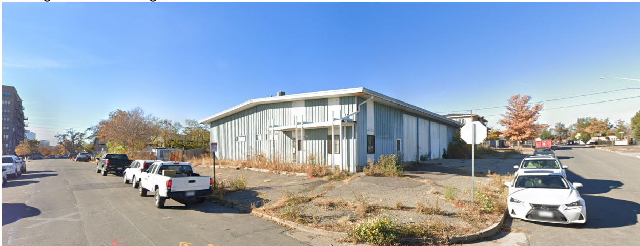
View of 4155 North Jason Street, looking southwest.
