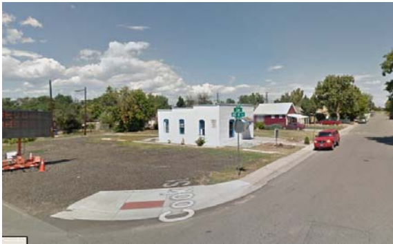
North – at 40 th Ave & Cook St.
