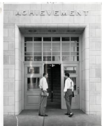
Welton St. entry to 1947 addition
