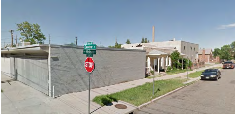
Corner of Decatur and Holden, looking northeast
