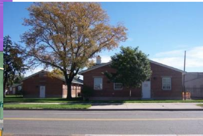
Inner City Health Center looking east
