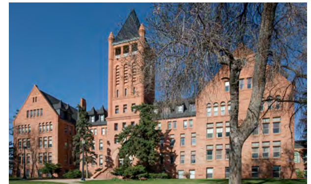
Top to bottom: Theater and Administration Building
