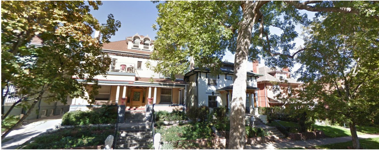
Three story single unit residential buildings west of the subject site, facing west from Race Street.
