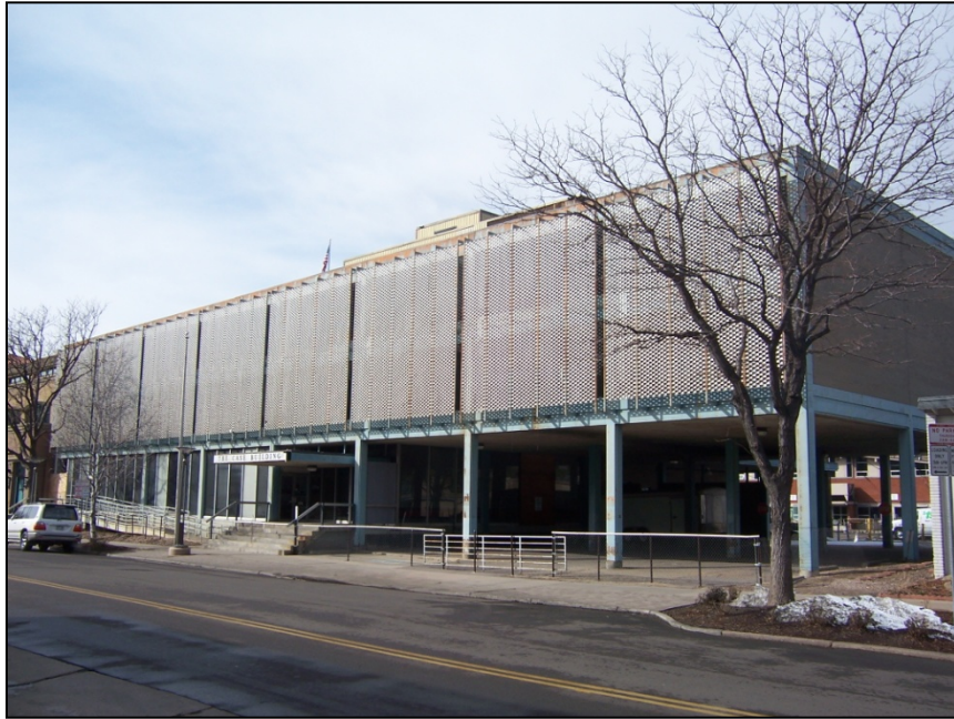
Existing building at 245 Columbine Street as viewed from Columbine Street.
