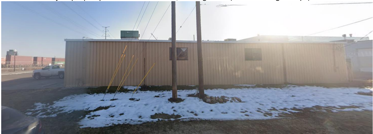
View of the subject property on W. 43 rd Avenue, looking south. (Source: Google Maps)
