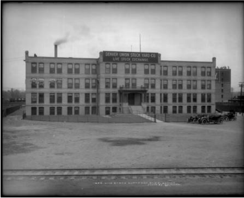
Figure B-1. 1908 photo of the 1898 Livestock Exchange structure showing the original facade, portico, and corner finials. 80
