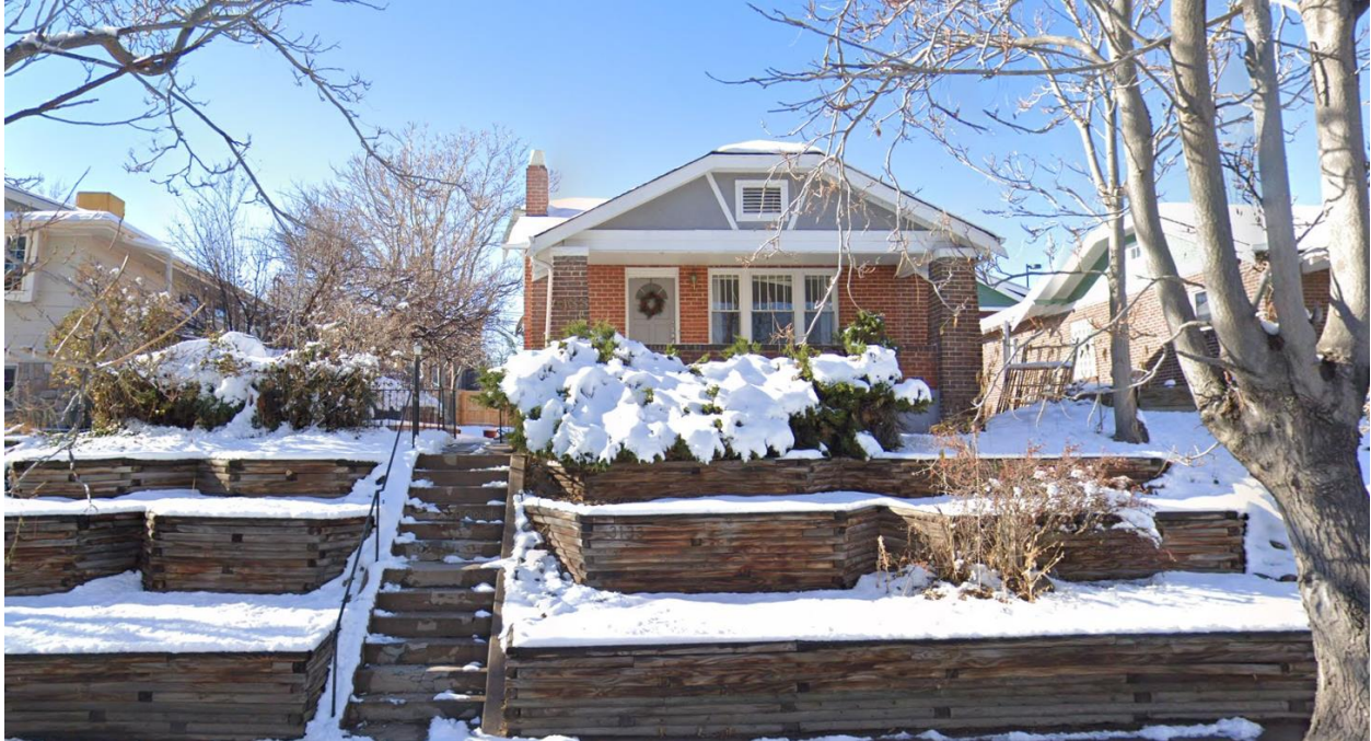
View of subject property looking west.
