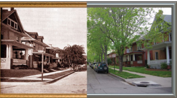
14th Avenue A, Frank S. Snell Subdivision Historic District. Historic photo on left 1911; current photo on right 2014.
