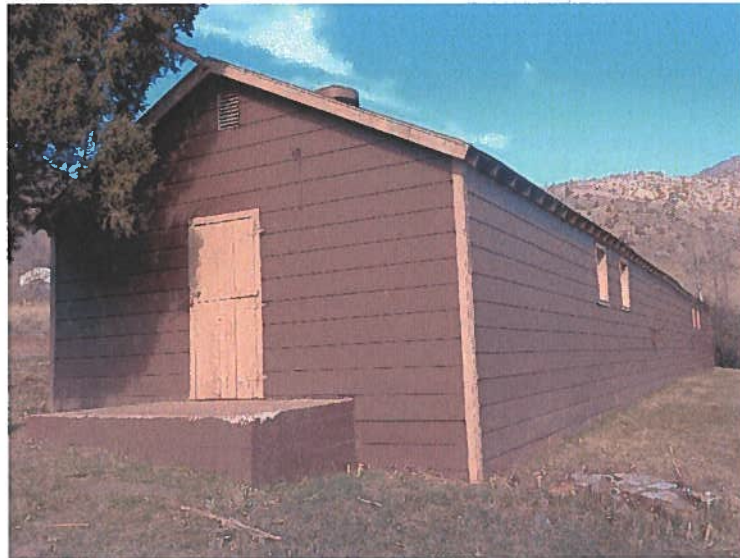
East and north elevations of Building 1
