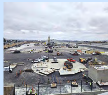
Construction photos courtesy of San Diego International Airport
