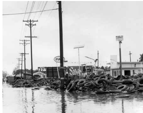
Damage from flooding, June 1965.
