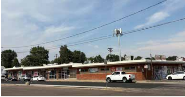
Many shopping centers house local businesses and services.
