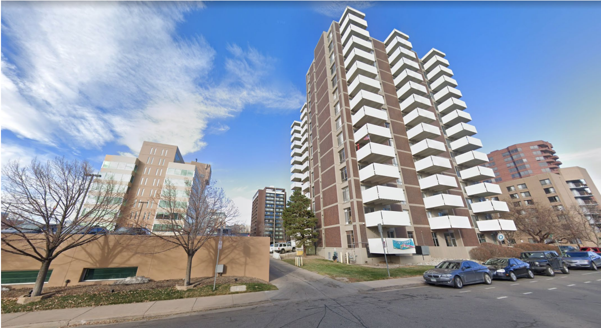
Site – from Ellsworth Avenue, facing north
