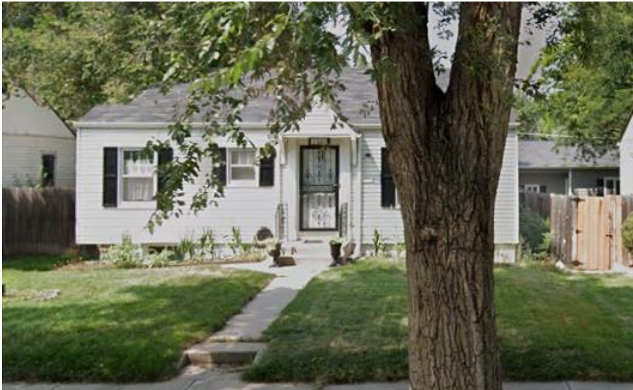
View of the property to the west across S. Gilpin St., looking west.
