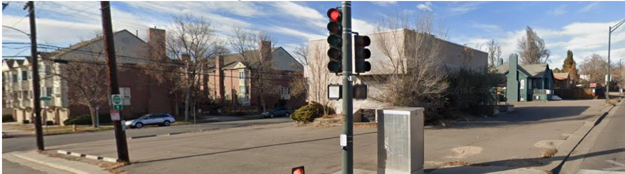
Above: Site-65 and 55 S. Colorado Blvd. – looking northwest from S. Colorado Blvd. and Bayaud Ave.
