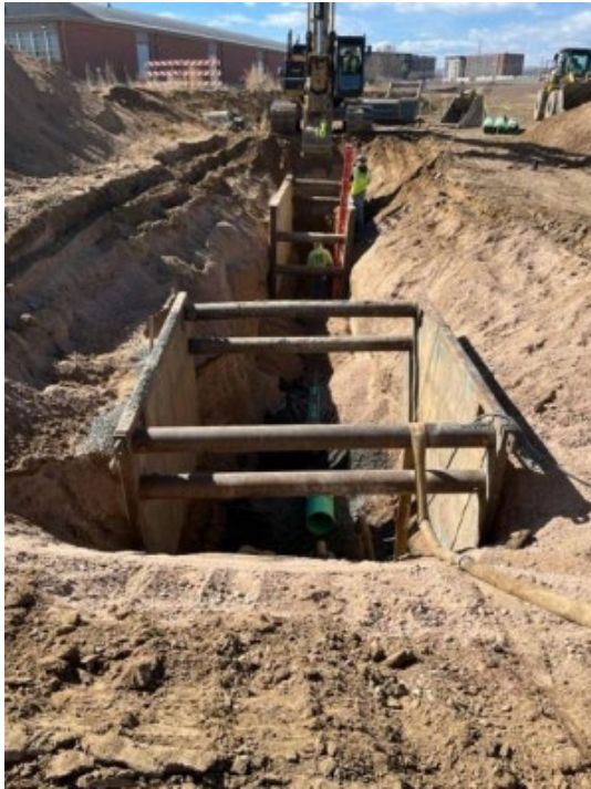
Sanitary Sewer Pipe Installation
