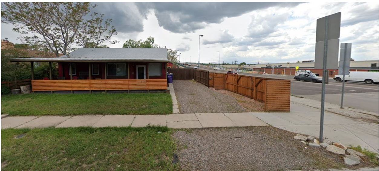
South – from South Bannock Street (Source: Google Maps)
