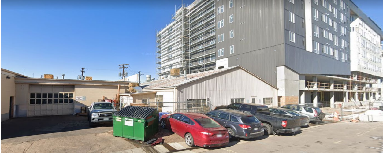
West – from South Cherokee Street (Source: Google Maps)
