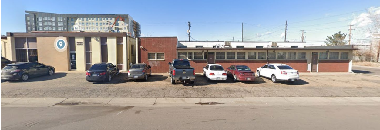
North – from South Bannock Street (Source: Google Maps)
