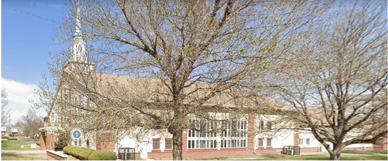
Place of worship west of the subject property across Colorado Blvd., looking west.
