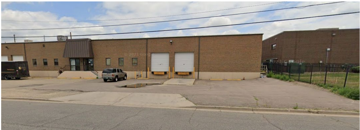
Industrial warehouses east of subject property, looking east.
