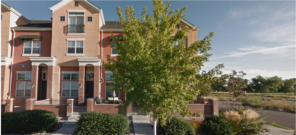
Multi-unit residential directly north of subject property, looking north from the internal private roadway serving the development.
