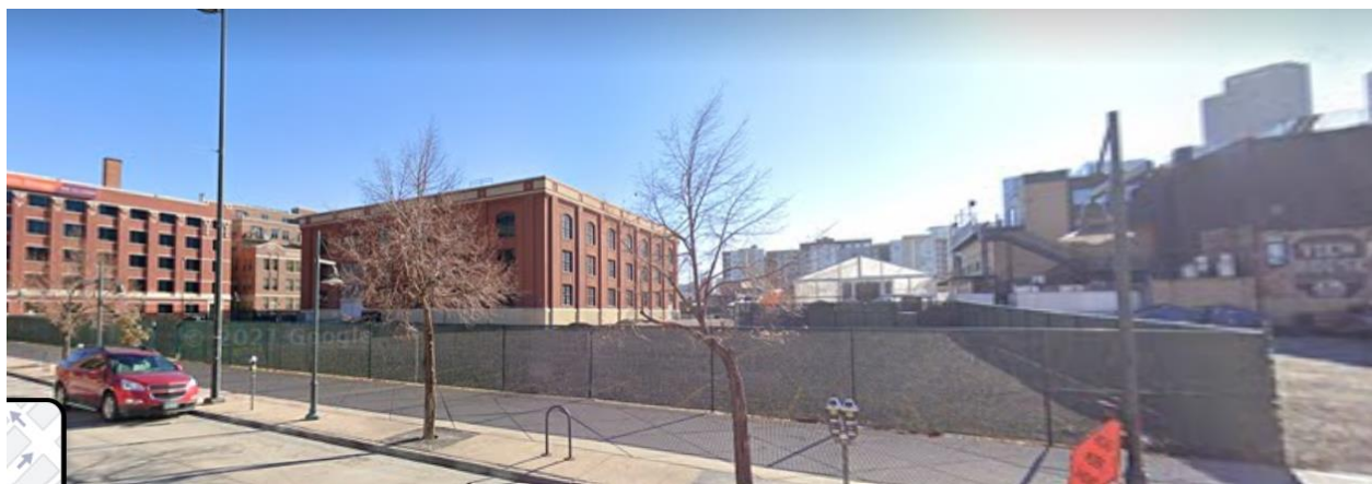
View of surface parking and other nearby development north and east of the subject site (Google Maps)
