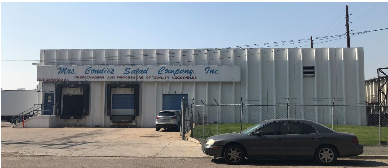
Site - Looking west from Denargo Street
