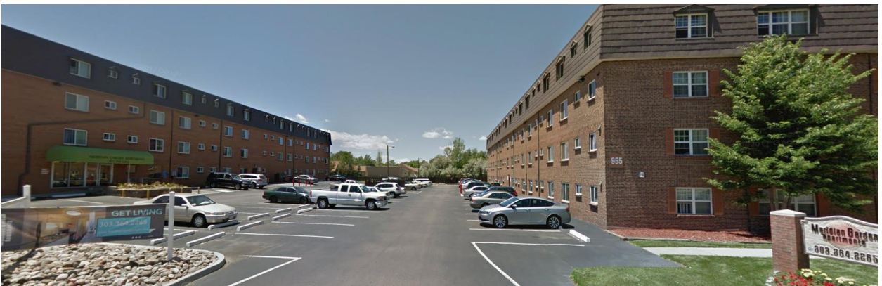
Four-story multi-unit residential buildings east of the subject property facing west from South Havana Street.
