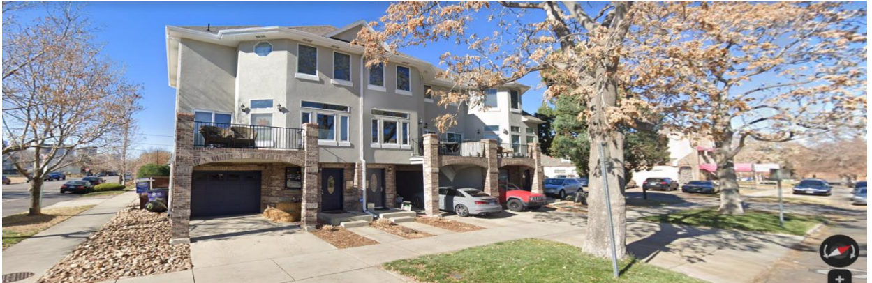
View of townhouse development to the south of the subject property, looking northwest from N. Ogden St.
