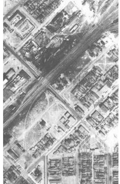
1933 aerial image showing the convergence of Downing, Blake, Lafayette and 38th streets near the Union Pacific rail corridor.
