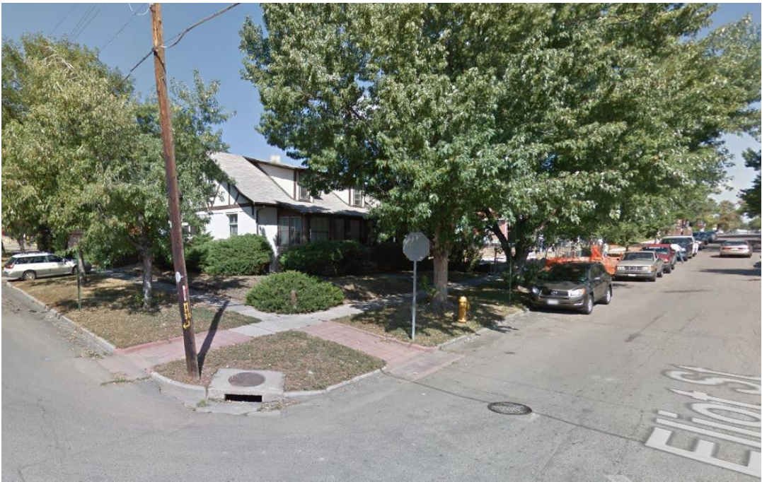
Subject Site, looking northwest
