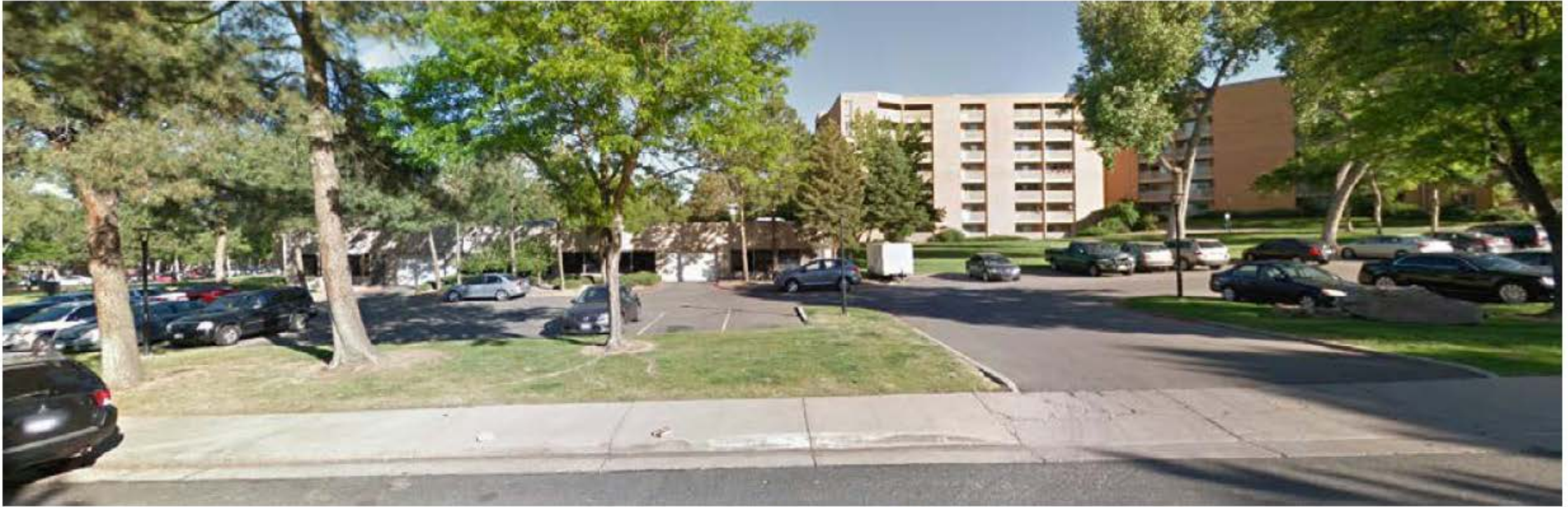
Woodstream Village Looking West
