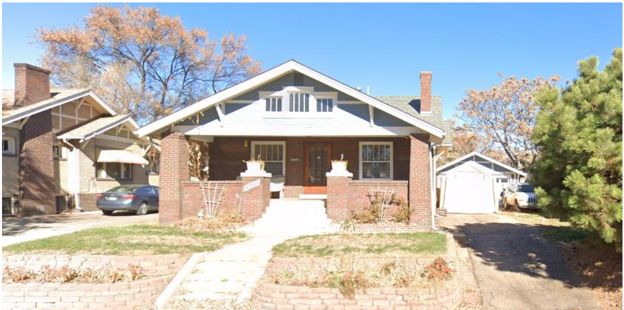
View of the property to the west, looking north.
