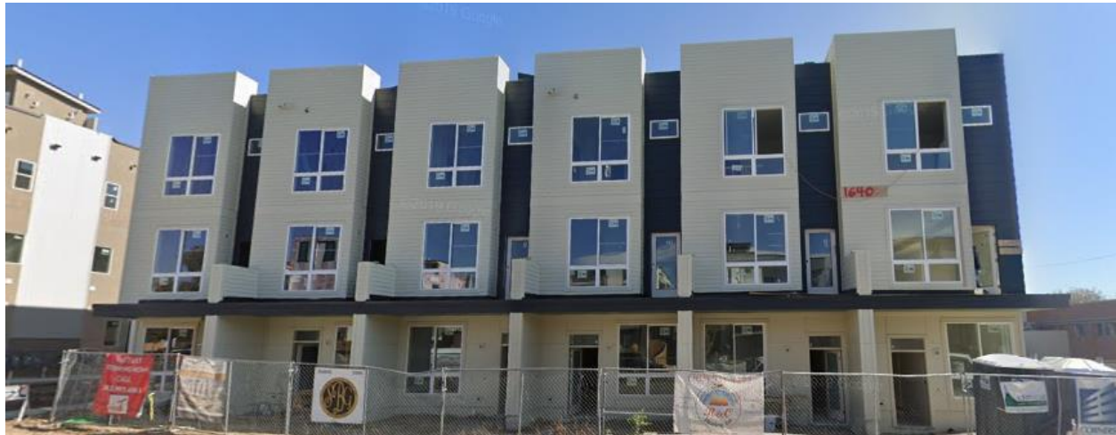
Three-story multi-unit residential building north of the subject site, facing east from Julian Street.
