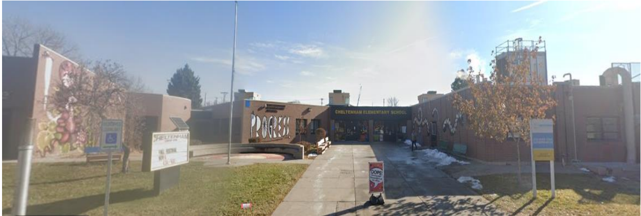
Single-story, elementary school building directly south of the subject site, facing east from Julian Street.
