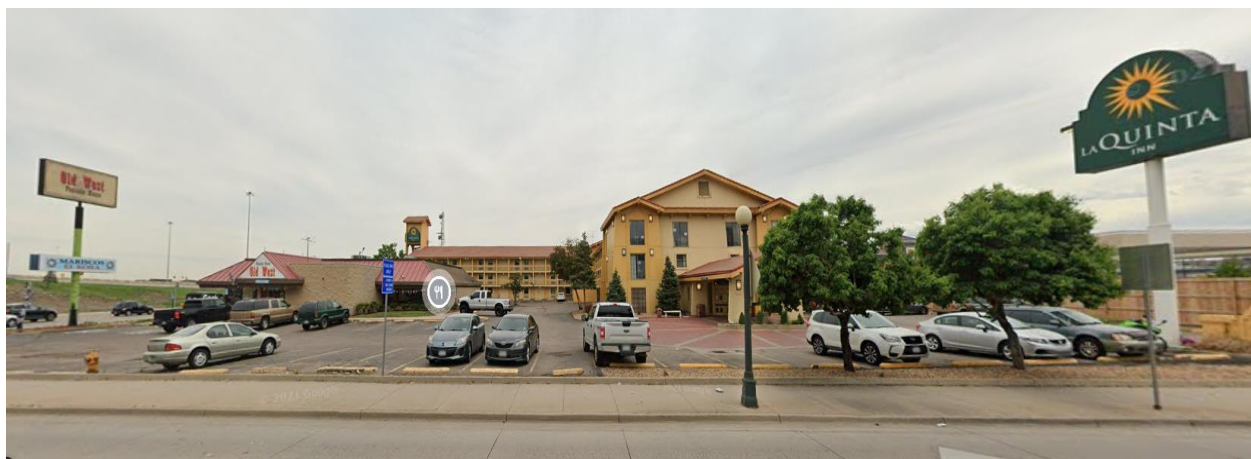
View of the subject properties, looking east.
