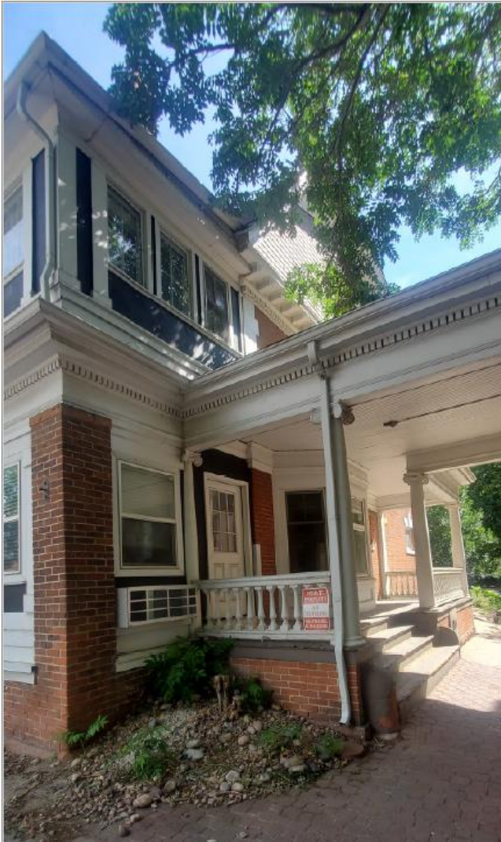
Southwest corner showing car port and entrance.
