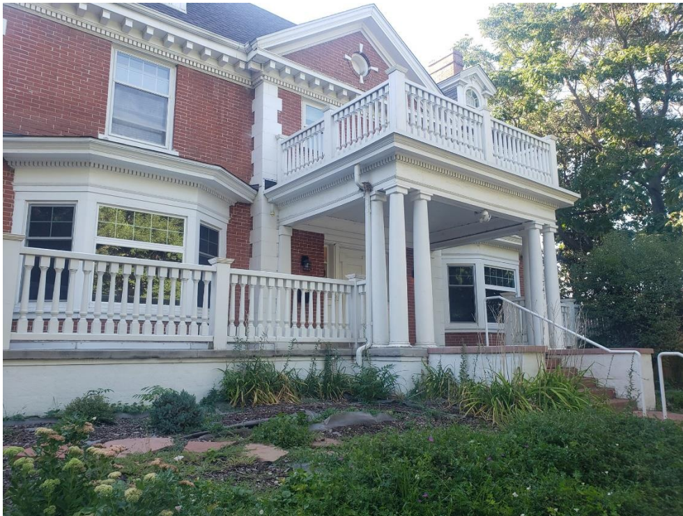
Street level, east side, close up.
