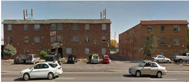
Low-rise multi-units north of the subject property
