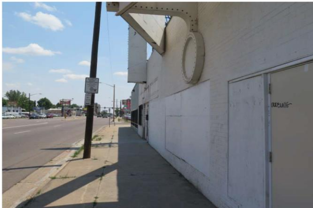
Boarded windows and doors
