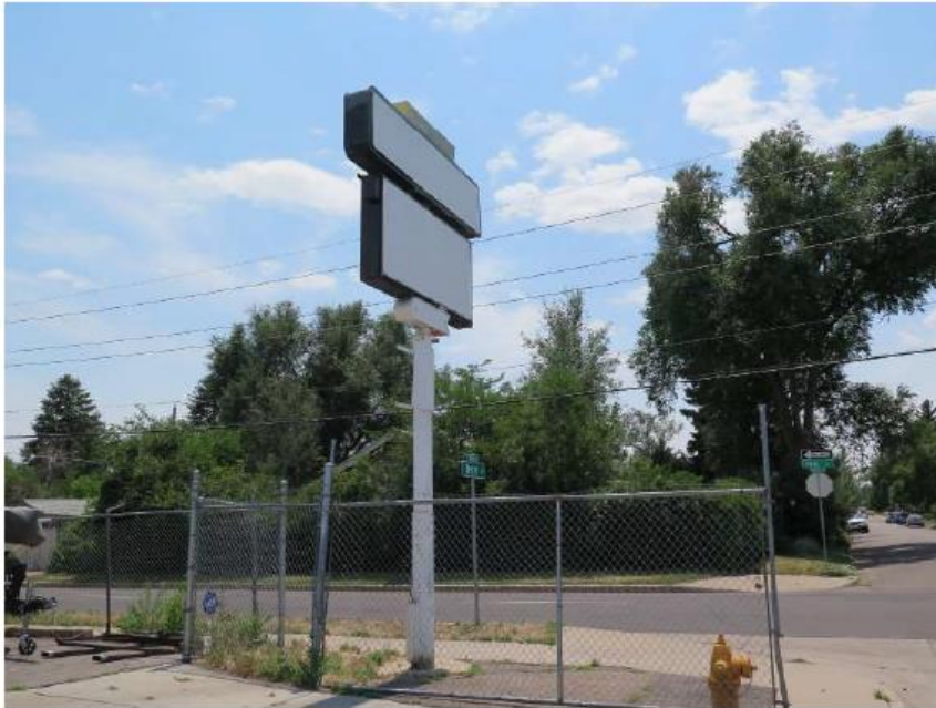
Numerous blank signs were noted
