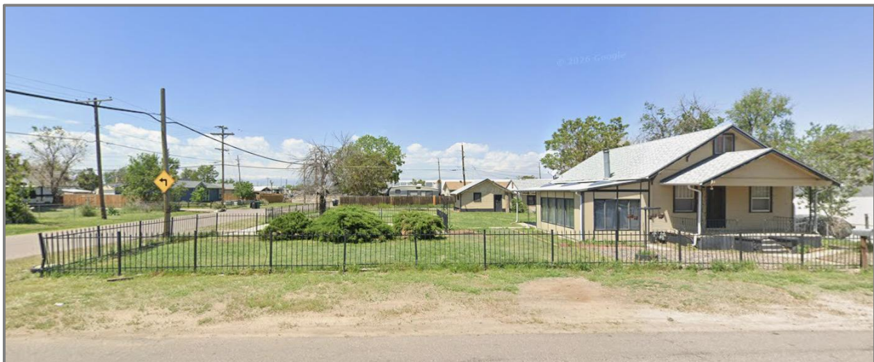
View of the subject property looking west from North Milwaukee Street.
