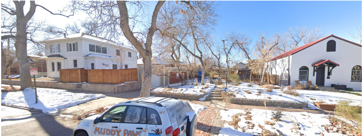
View of the property to the north, looking west.
