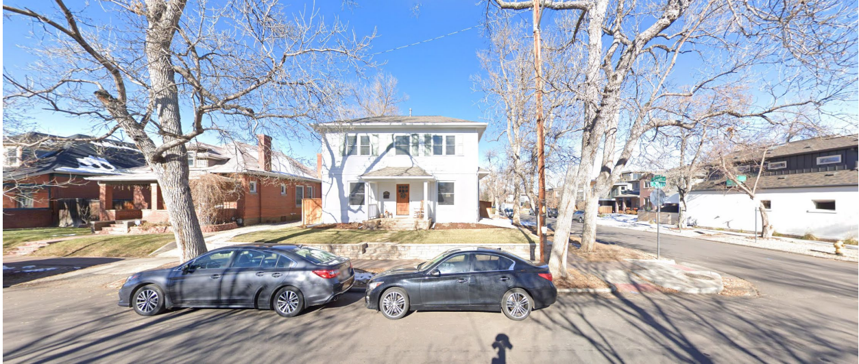
View of the subject property, looking north.
