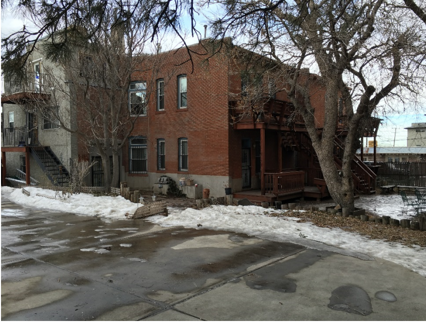
West Elevation of the Cole Apartment Building
