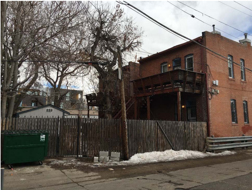
South Elevation of the Cole Apartment Building
