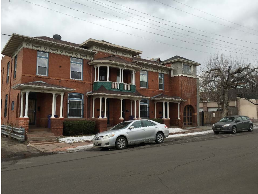
North Elevation of the Cole Apartment Building
