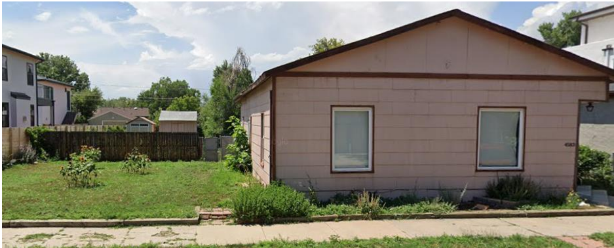
Subject Property - View of 4583 North Yates Street, looking west.
