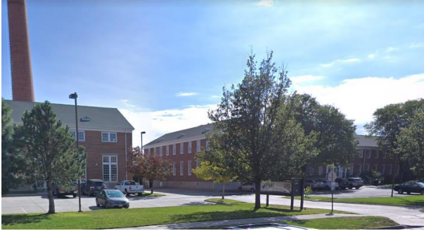
Northern portion of Subject Property
